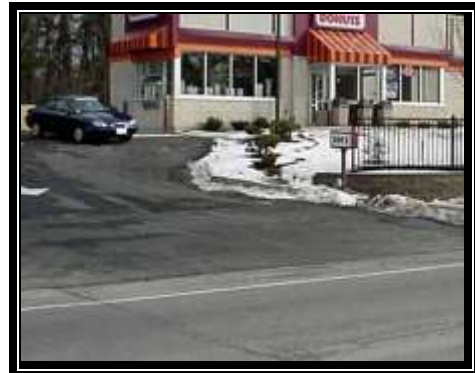
Inappropriate leveling area
