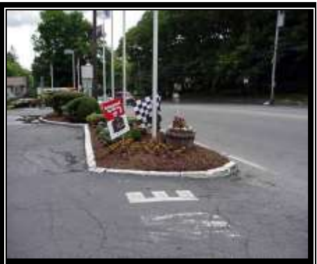
Inappropriate separation from road
